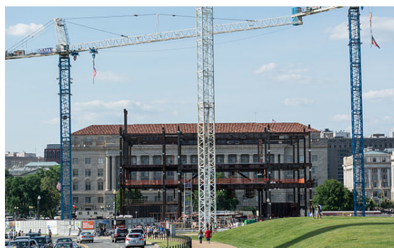
The museum under construction in May 2014.
