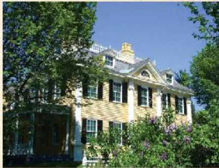
JOHN VASSALL HOUSE
